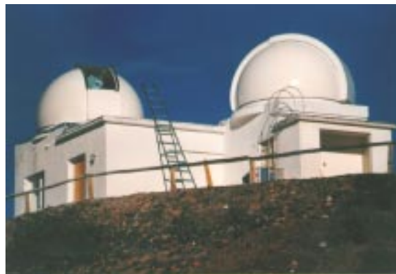
MICA and HASTA building.
